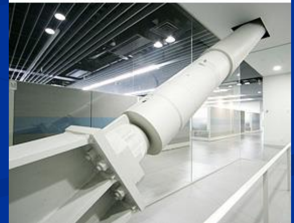
Seismic damper system absorbs earthquake vibrations
