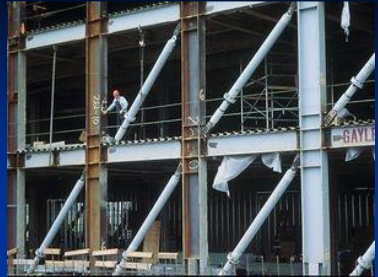
Seismic damper system absorbs earthquake vibrations
