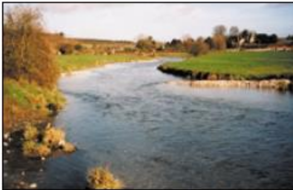
Groynes in place already increasing flow diversity
